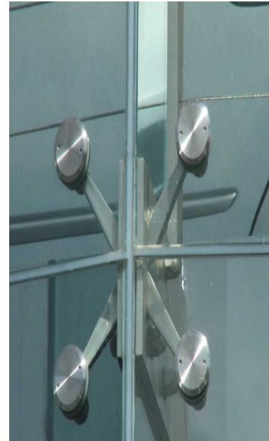
Figure 3 - Point Fix Curtain Wall
