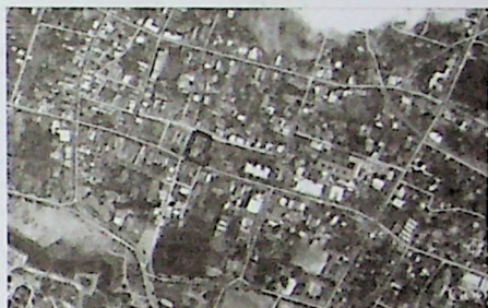
Figure: 37 – Constructing new linking roads and widening the existing Roads
