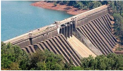
Fig. 10. Konya dam, India - 53 years, old
