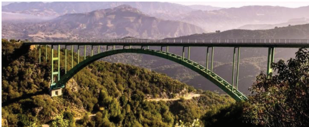
Fig. 7. Cold Canyon arch bridge
