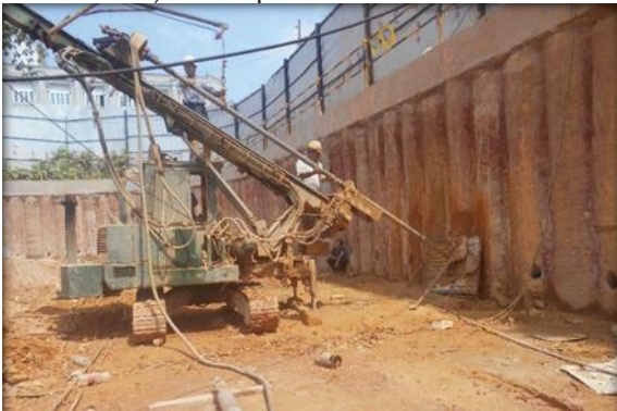
Figure 16 Drilling the Anchor hole
