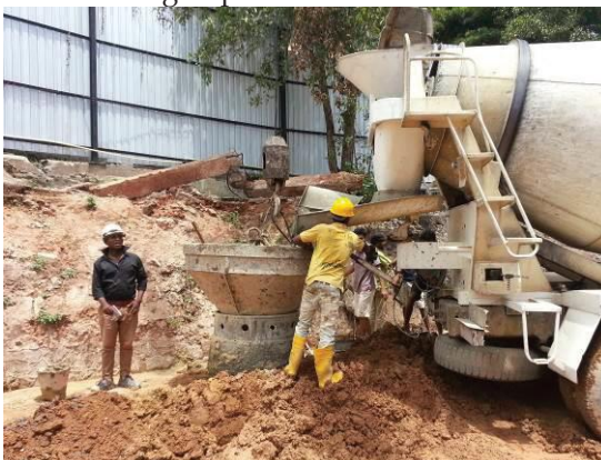
Figure 12 Concreting the Secant pile
