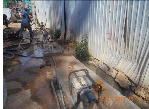
Figure 13 Pressure Grouting
