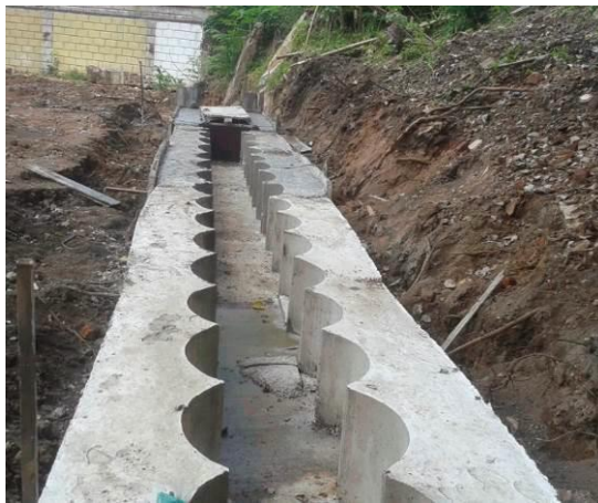
Figure 11 Concreted Guide wall
