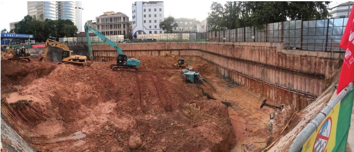
Figure 25 Secant Pile wall during excavation
