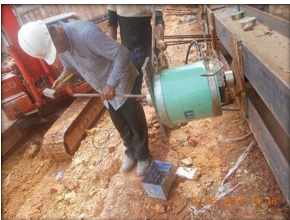
Figure 17 During GA stressing
