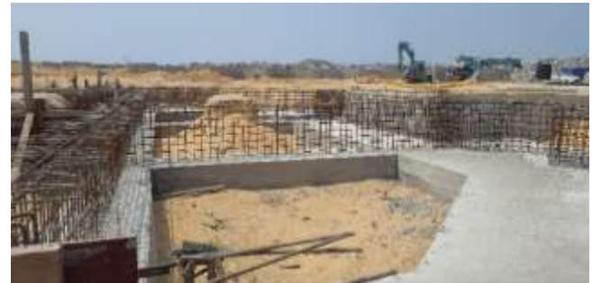
Figure 17: Strip foundation used to support the foundation.
