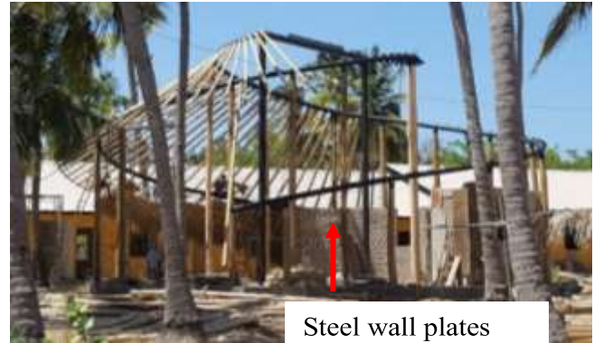
Figure 3: Steel and timber used in combination to form the complex structure.
