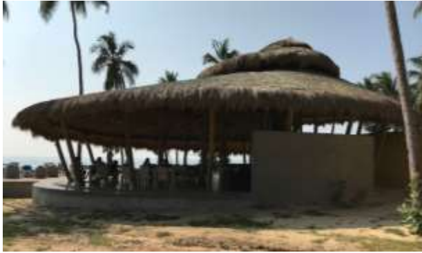
Figure 8: Completed form of a timber structure.
