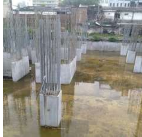
Figure 22: Existing columns to be strengthened
