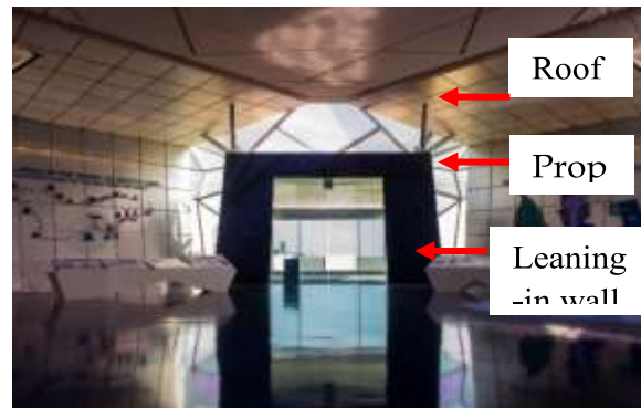
Figure 11: Structural elements of the pavilion.
