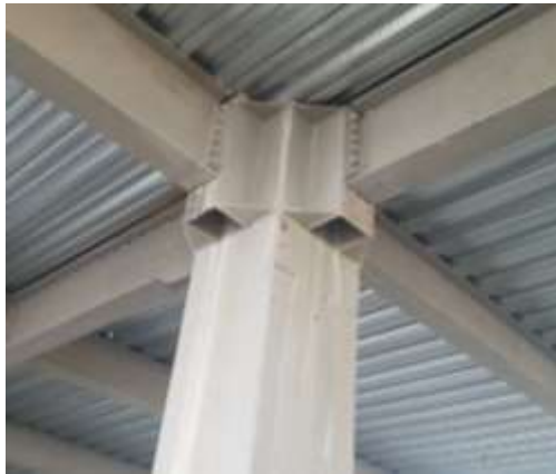
Figure 21: CFST column connection at floor.
