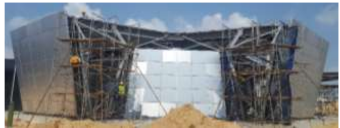
Figure 17: Unitized curtain wall system adopted to clad the structure
