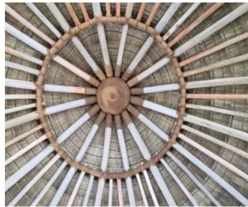
Figure 5: Connection of timber rafters at the ridge.
