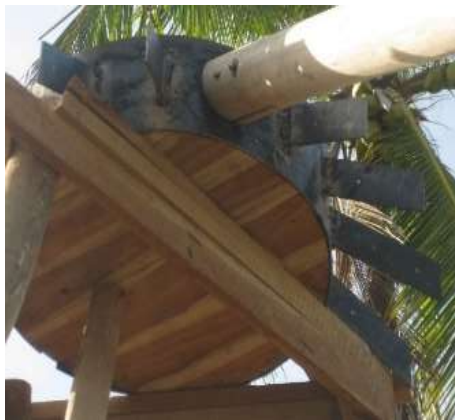
Figure 5: Connection of timber rafters at the ridge.
