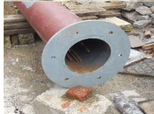
Figure 18: Base plate for CFST column.
