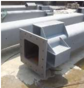
Figure 19: CFST column head detail at flat slab.
