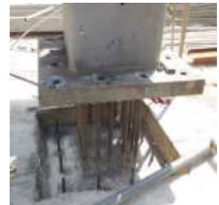
Figure 20: Base plate for CFST column.
