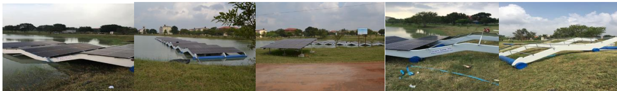
Figure 1: Floating Solar Plant at Kilinochchi Premises of the University of Jaffna
