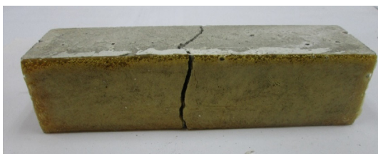
Fig. 14. The crack propagation of the test specimens on bottom face which contain PU layer on bottom face.
