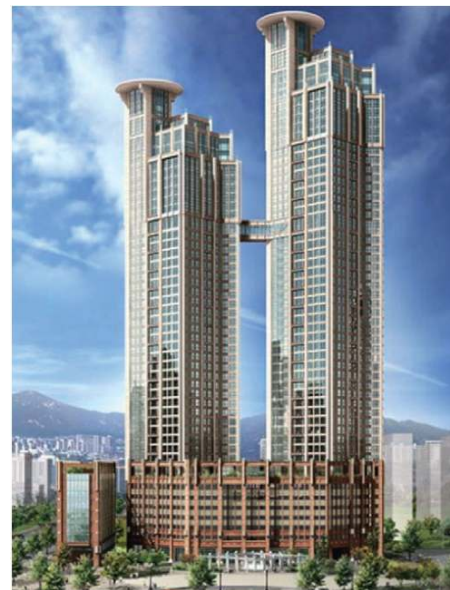
Figure 11. Tower in Seoul, Korea (Abada, 2004)
