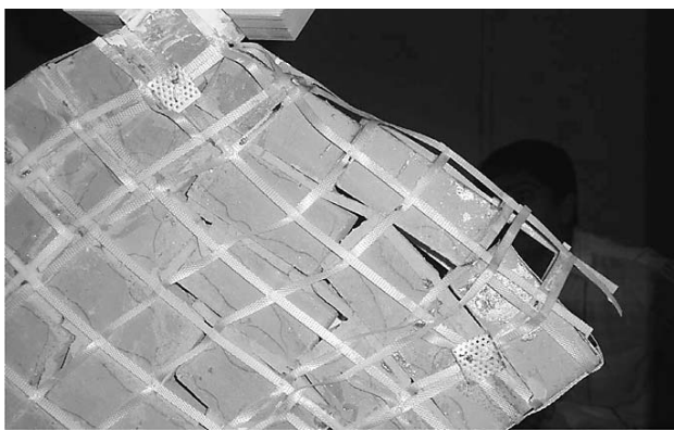
Fig. 6 Epoxy failure at top edge
