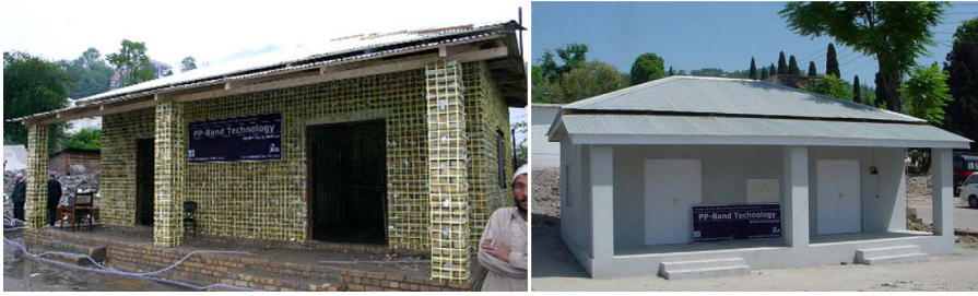
Figure 3. House in Pakistan retrofitted with PP-band mesh (JBIC 2007).
