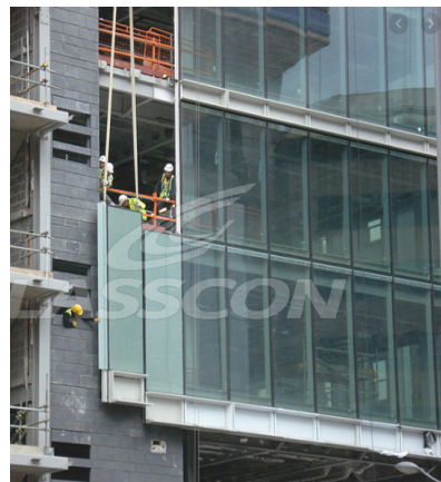
Figure 1:- Unitized curtain wall arrangement
