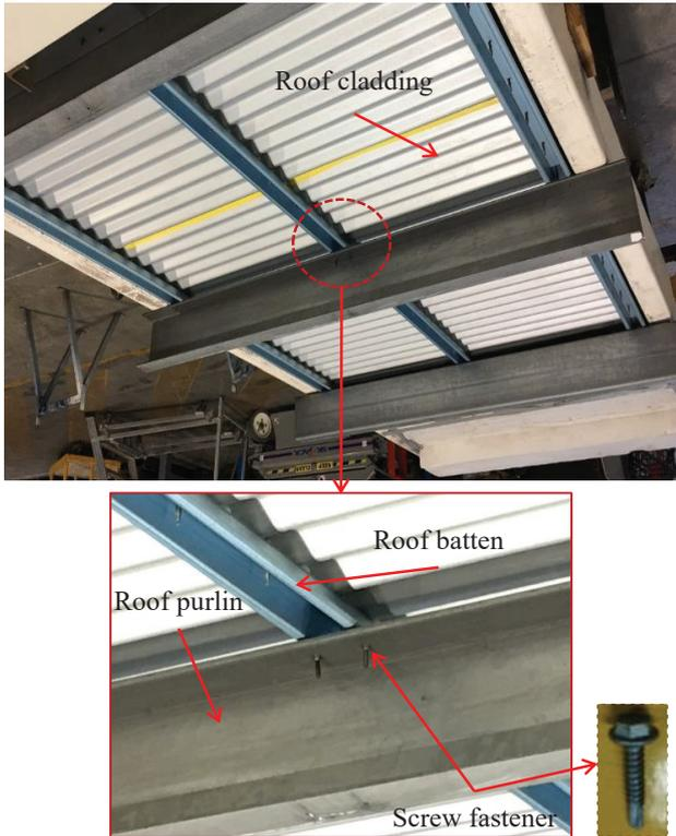
Fig. 1. Typical Thin Steel Roof Structure
